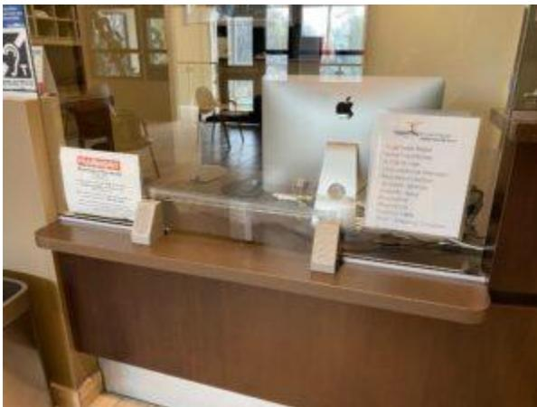
two STS-K002 systems were installed. The system features our STS-SU1 Staff Unit, which includes a switch to mute on the staff side, a patient side counter microphone and speaker, as well as a hearing loop antenna. The mute feature allows the administrative team to control the system with ease and ensure patient information confidentiality on their side of the partition. The hearing loop antenna makes it a hearing accessible space for
